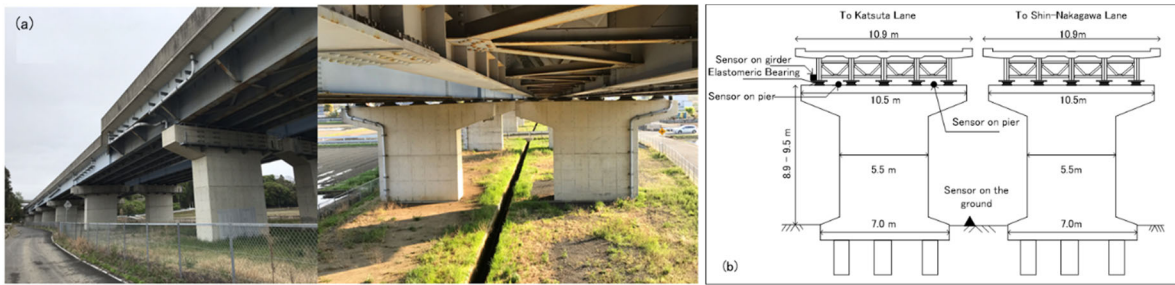
Fig. 3. Katsuta Highway multi-span viaduct (a) Photos (b) Dimension.
