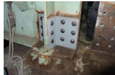
Figure 1. An example of the repair with high-strength bolts
