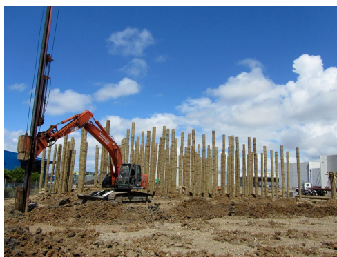
図-12 中大径木の施工状況: New Zealand (TTT Products Limited)
