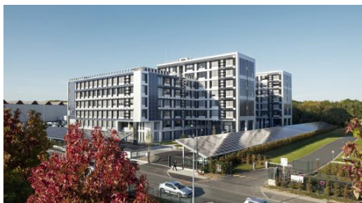
写真-5 Green Office Meudon
