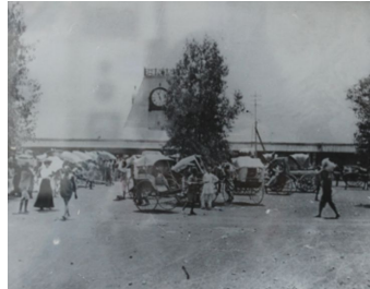
図1 Nairobi Railway Station 1900
