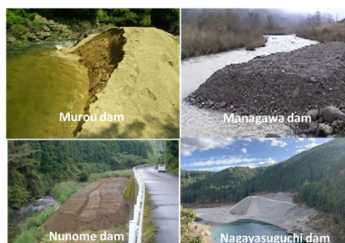
Fig. 2: Examples of SR stockpiles in Japan, including the target study area in Naka River, Tokushima.
