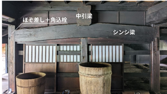
Figure 4 補強対象架構
