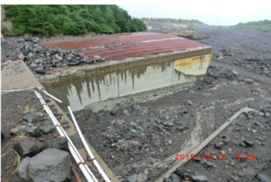
Figure 4. Screen dam located in Nojiri-River, Sakurajima
