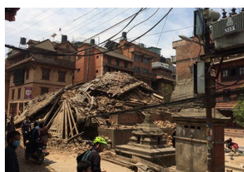
Photo.6 Collapse of Kurishna Temple
