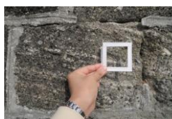
塀（凝灰岩）5400ppm
