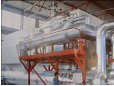
Fig.6 Hotwater Pipelines from Beznau nuclear power plant (NOK/REFUNA)[5]
