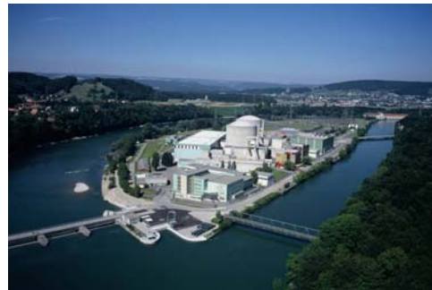
Fig.5 Beznau nuclear power plant and hot-water pipelines[5]
