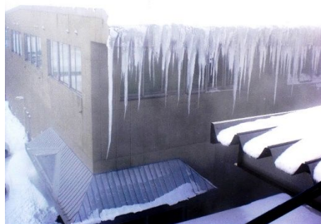
Fig. 1 Icicles at the edge of the folded-plate roof.
