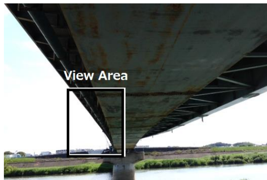
(a) Sakae bridge
