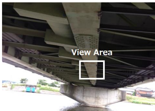
(b) Small bridge
