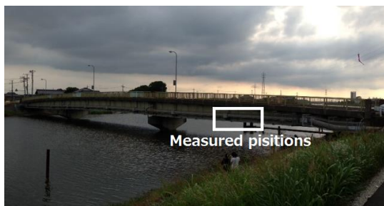
(b) Small bridge
