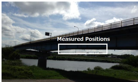
(a) Sakae Bridge
